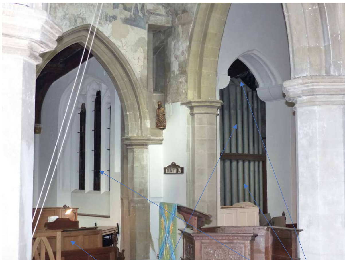
This shows the back of the 1939 console, the openings to Nave and Chancel, and the basses of the 16ft Geigen/Gamba, which are heavily mitred at the top.
